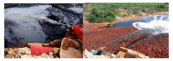
Figure 10. Sludge being washed-down with high-pressure wastewater
