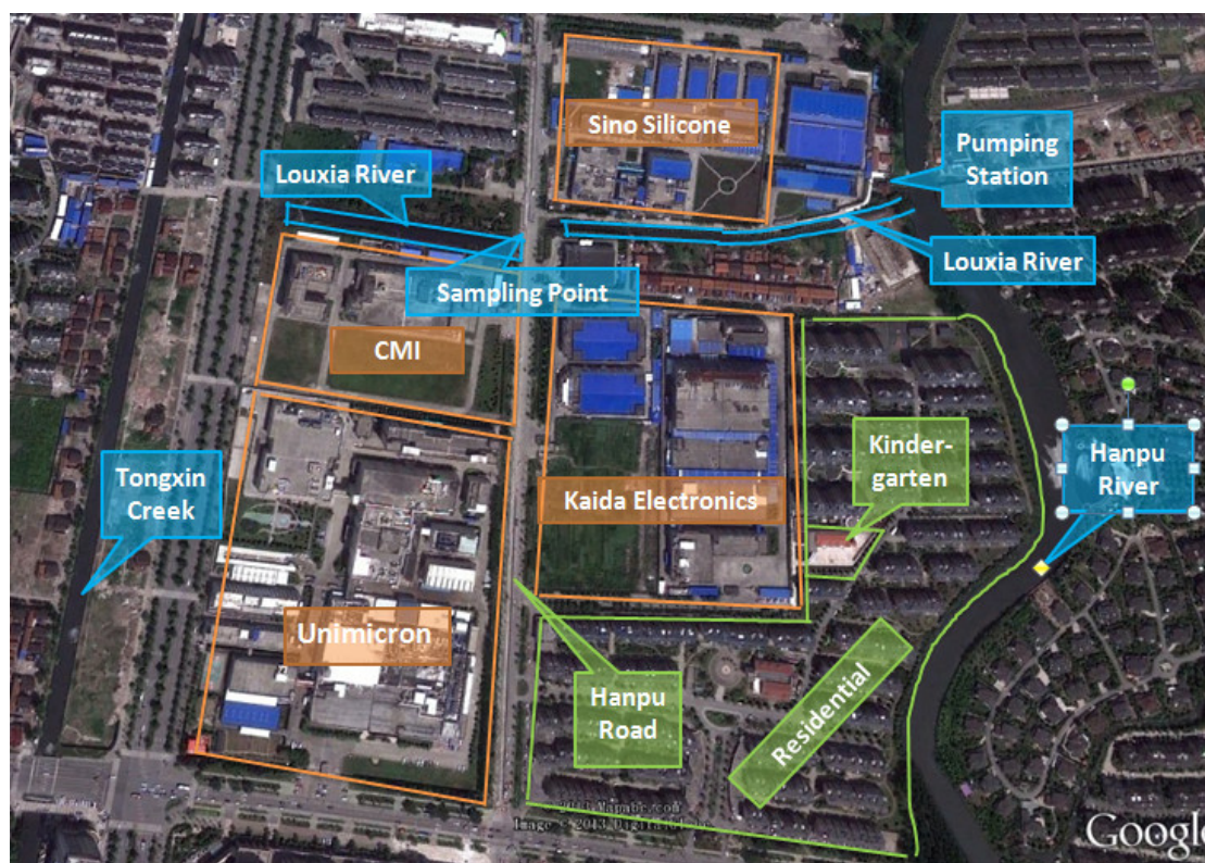
Figure 18. Factories and communities on the banks of the Louxia and Hanpu Rivers
