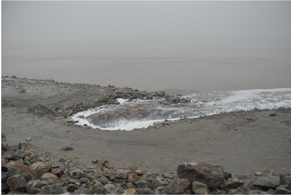
Figure 28 - Xiaoshan Linjiang Wastewater Treatment Plant discharge outlet. Photo: Lvse Jiangnan
