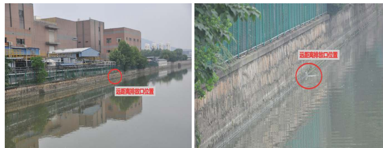
Figure 7. Location of hidden pipe
