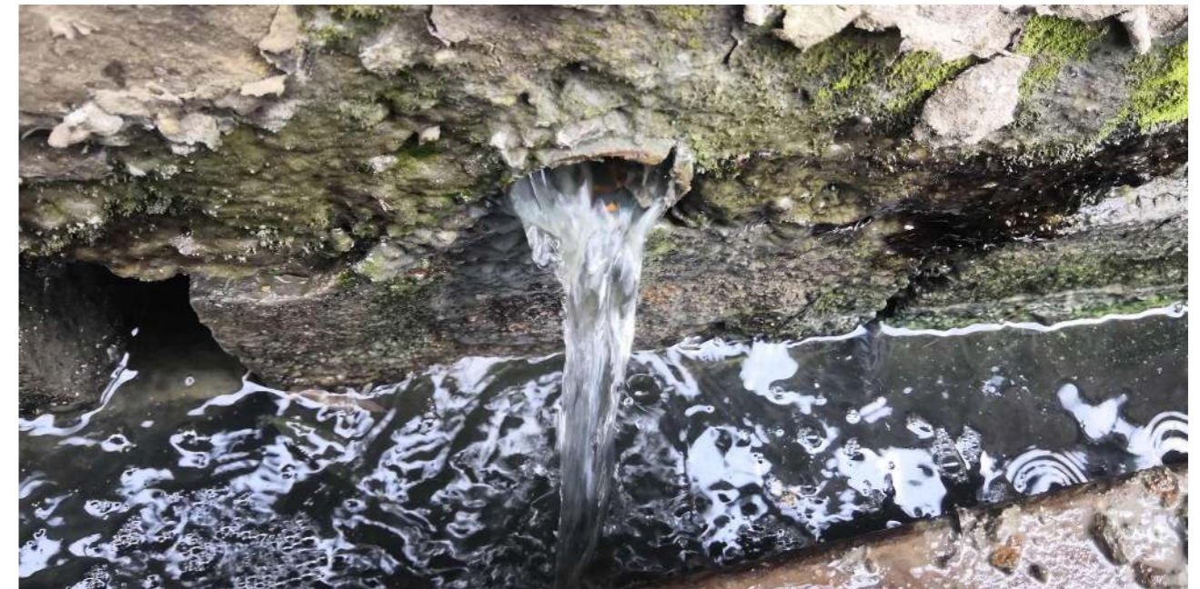
Figure 8. Lüse Jiangnan staff found this pipe discharging water
