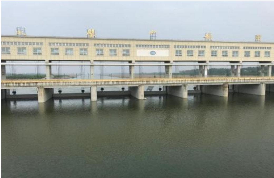
Fig. 27 Lingbi control gate
