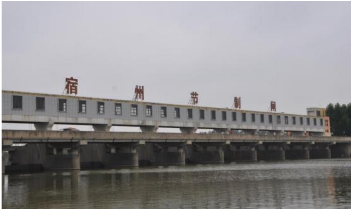
Fig. 37 Suzhou control gate
