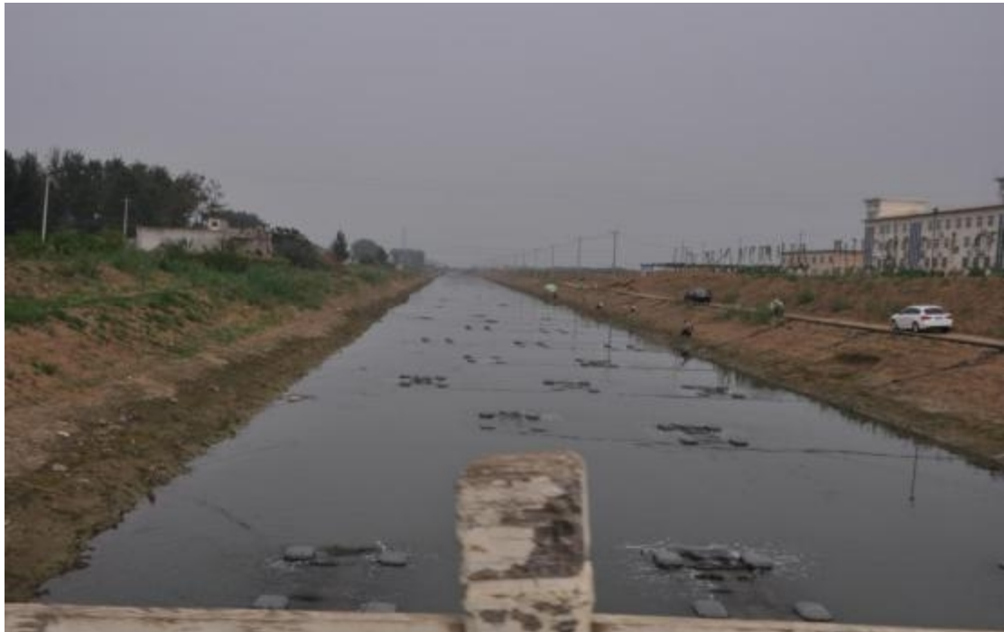
Fig. 26 Smelly waterways are densely populated with oxygen burst facilities that are being oxygenated.
