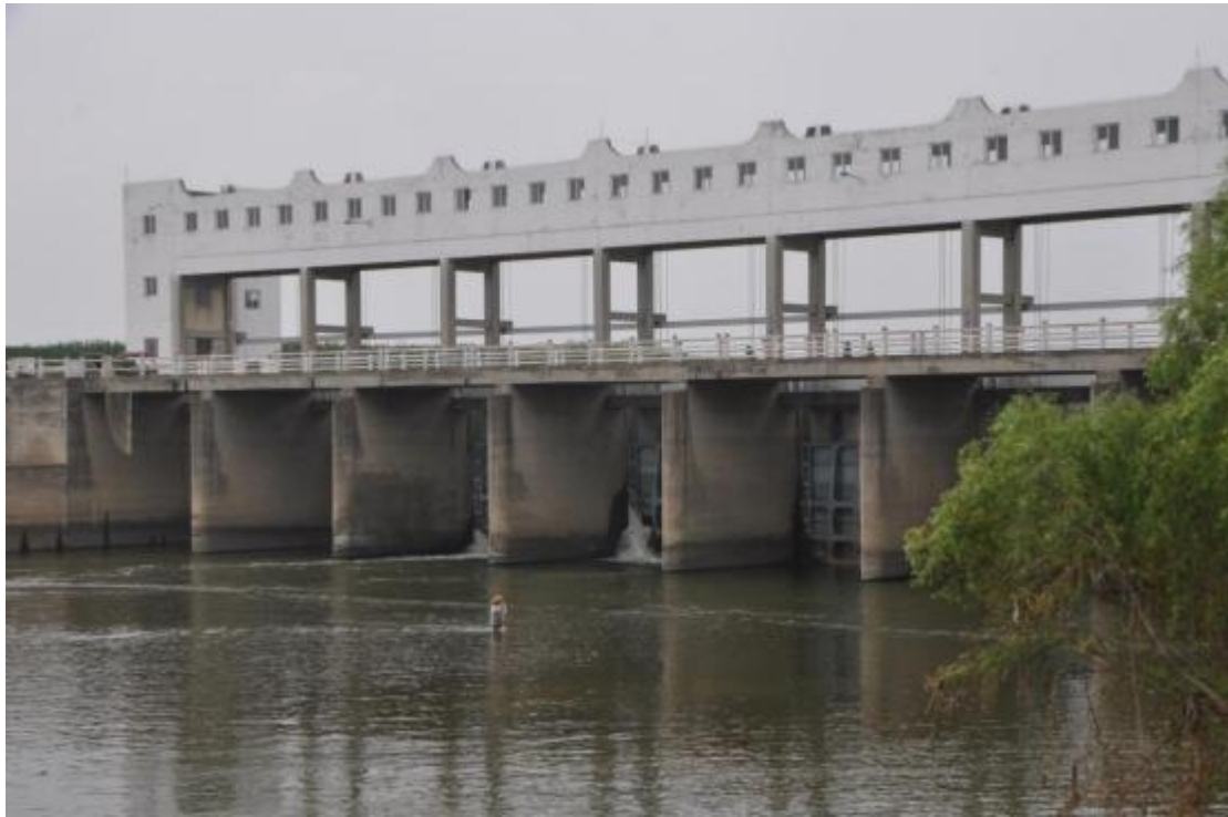
Fig. 13 The Kuhe gate is being lifted to release water.
