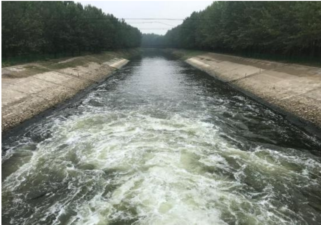
Fig. 41 Huangqiao gate being discharged
