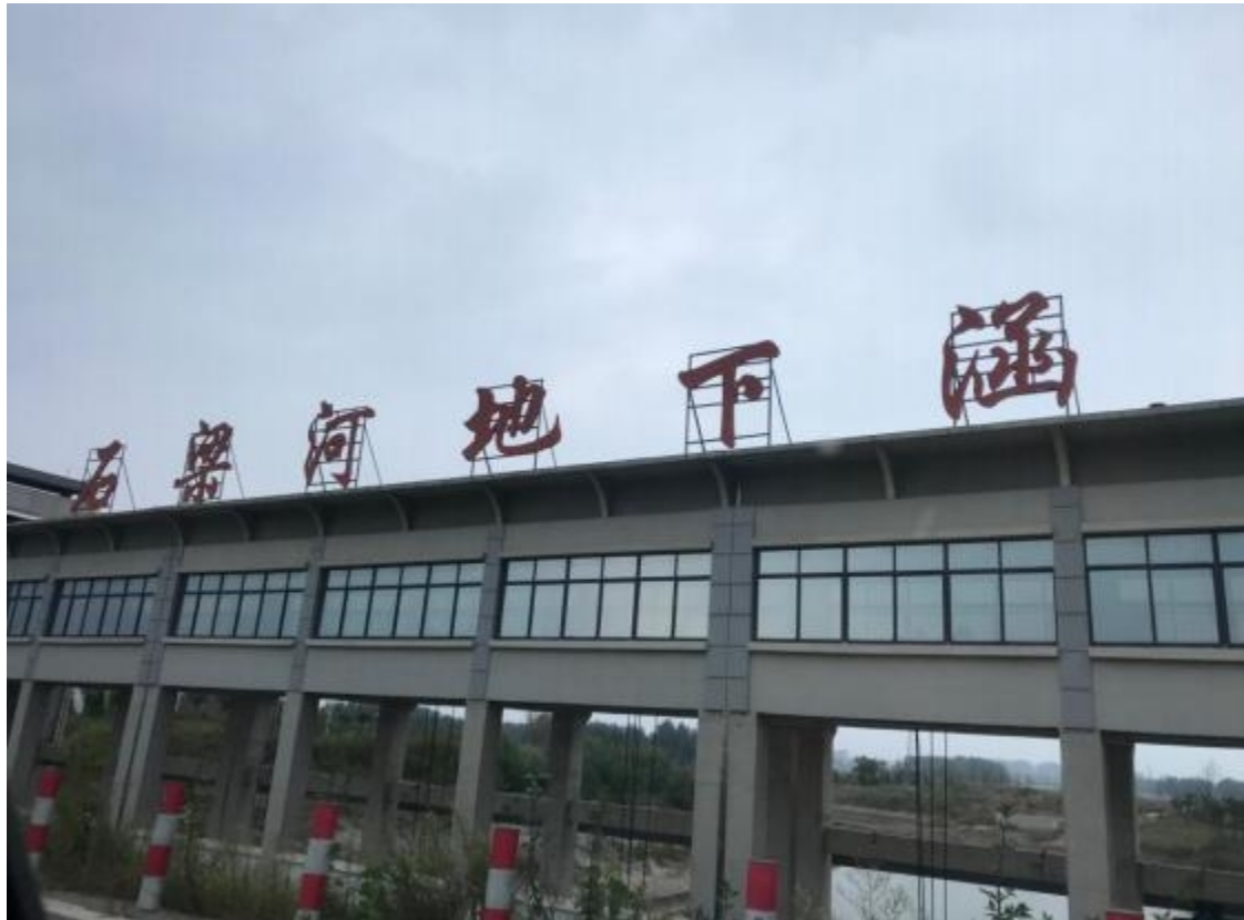
Fig. 21 The underground culvert gate of Shiliang River
