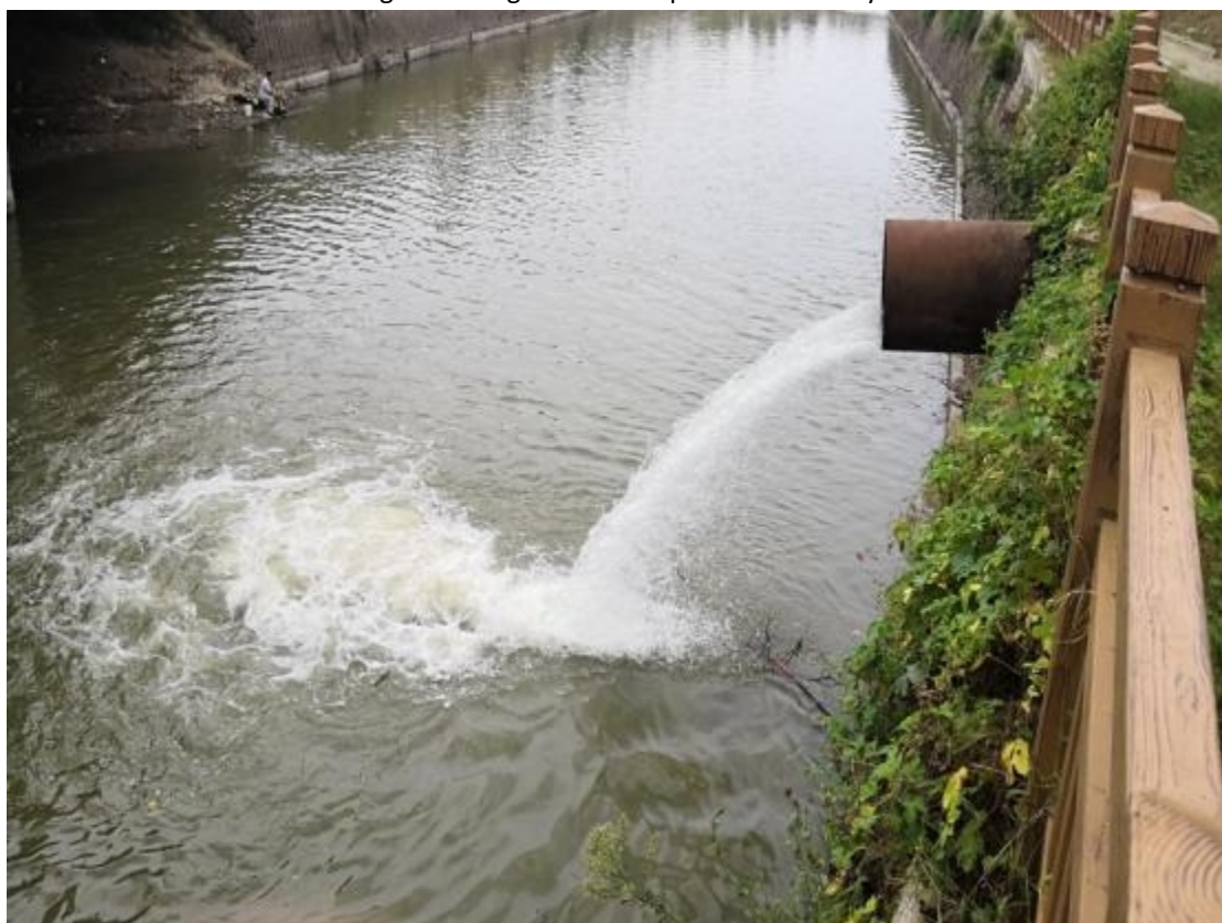
Fig. 18 The sewage outlet of the sewage treatment plant is draining water.
