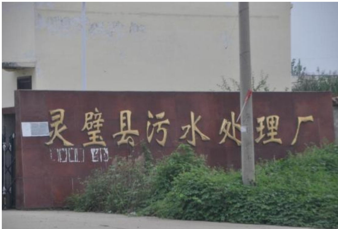
Fig. 24 Lingbi sewage treatment plant
