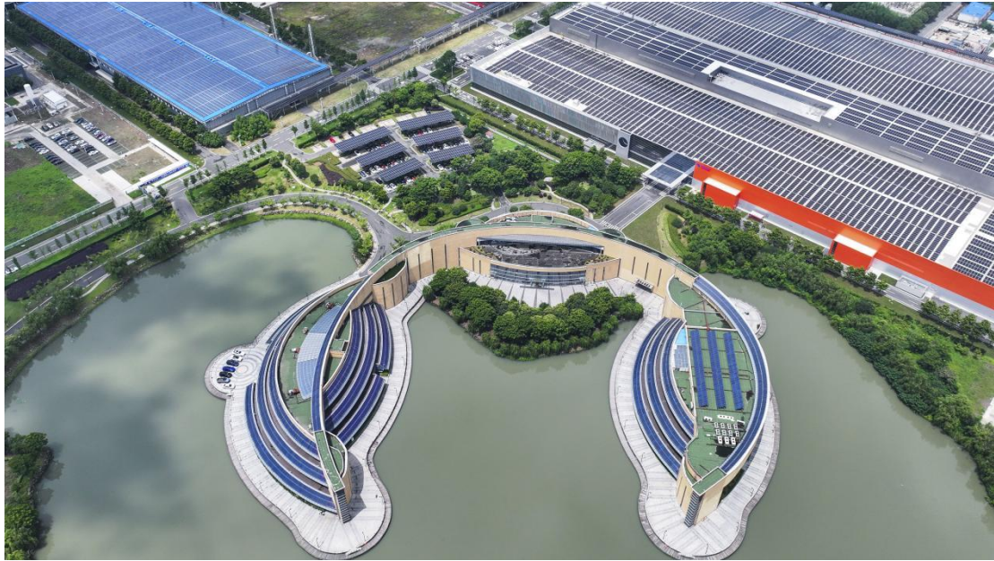
Figure 18 a photovoltaic company (photographed by PECC in July 2023)
