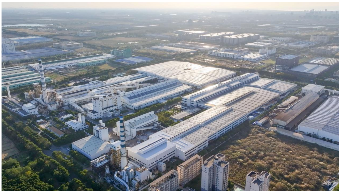
Figure 19 a photovoltaic company (photographed by PECC in November 2024)
