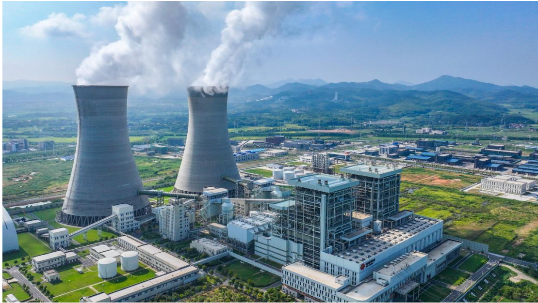
Figure 17 a thermal power plant (photographed by PECC in September 2024)
