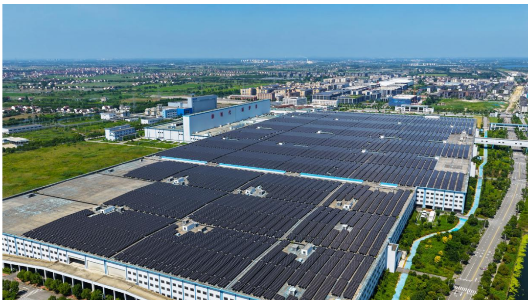
Figure 6 Futong Group Yangtze River Delta Information Technology Industrial Park (Photographed by PECC)
