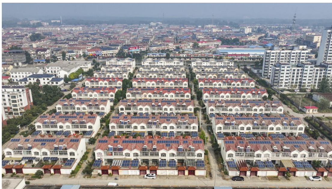
Figure 8 Qingnan Village in Lianyungang - Zero-Carbon Village (Photographed by PECC)
